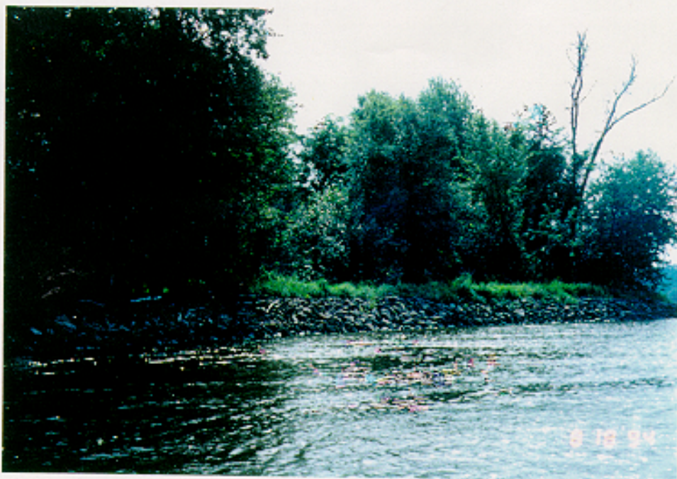
Photo #8 - Downstream end of riprap protection wing at closing structure, riprap soundly intact; August 1994
