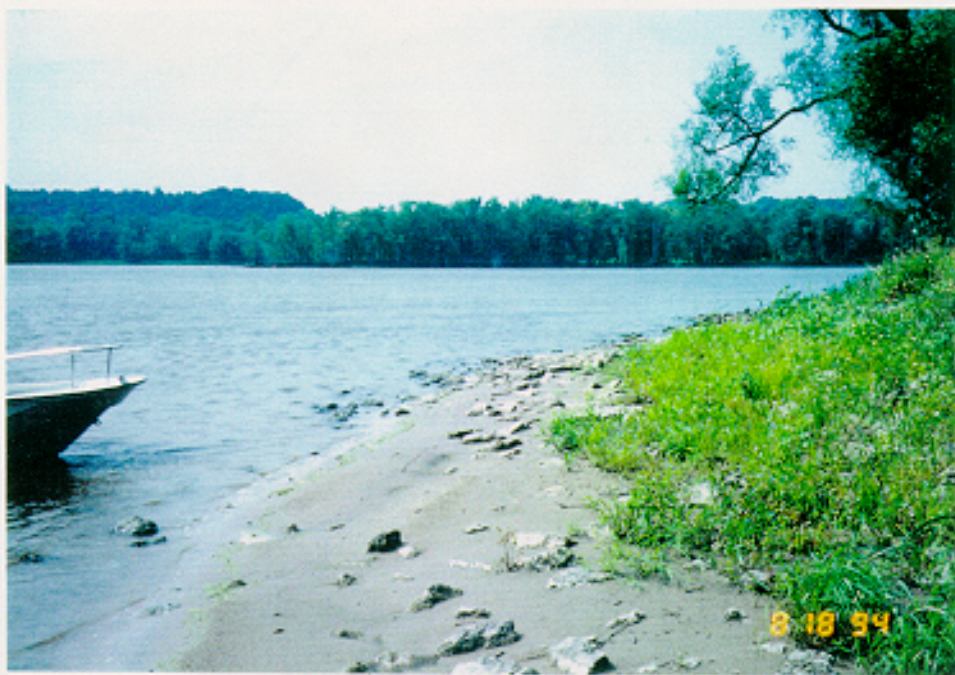
Photo #7 - Upstream end of riprap protection wing at closing structure, riprap washed away during flood of 1993; August 1994
